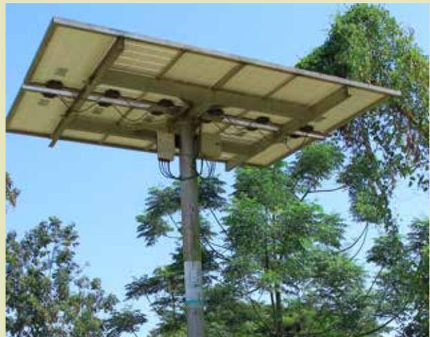
*Solar powered water pump panel*
